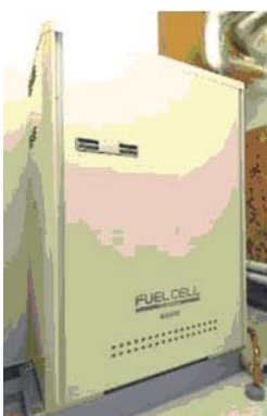
A Hokkaido Gas fuel cell Installed at a customers house (picture courtesy of Hokkaido Gas)
