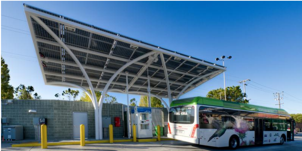
A fuel cell bus refuels at the Emeryville hydrogen station (Source: AC Transit)
