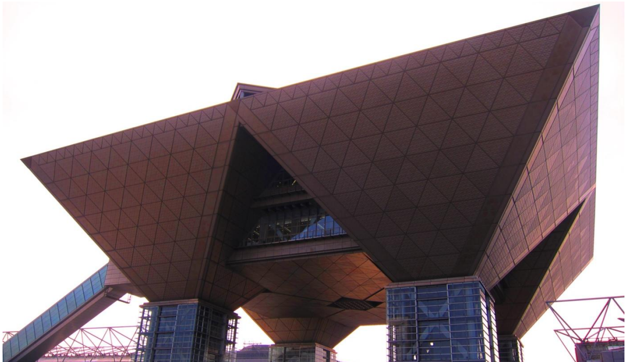
Tokyo Big Sight (Source: Jonathan Wing, Fuel Cell Today)
